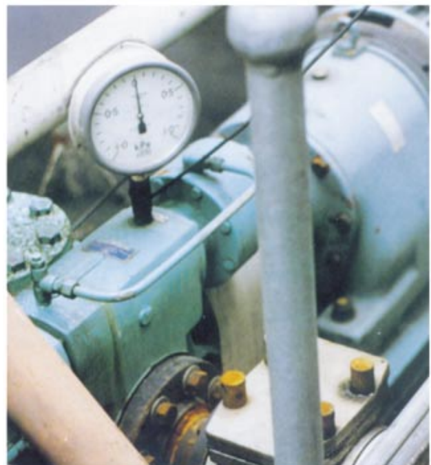
PFM Valve fitted to V40 Pump
